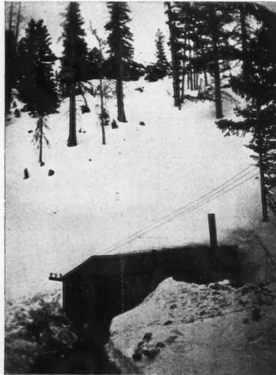
2. ENTRANCE TO TURKEY CREEK TUNNEL.
